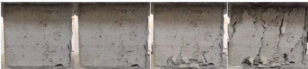
(c) Longitudinal splitting failure
